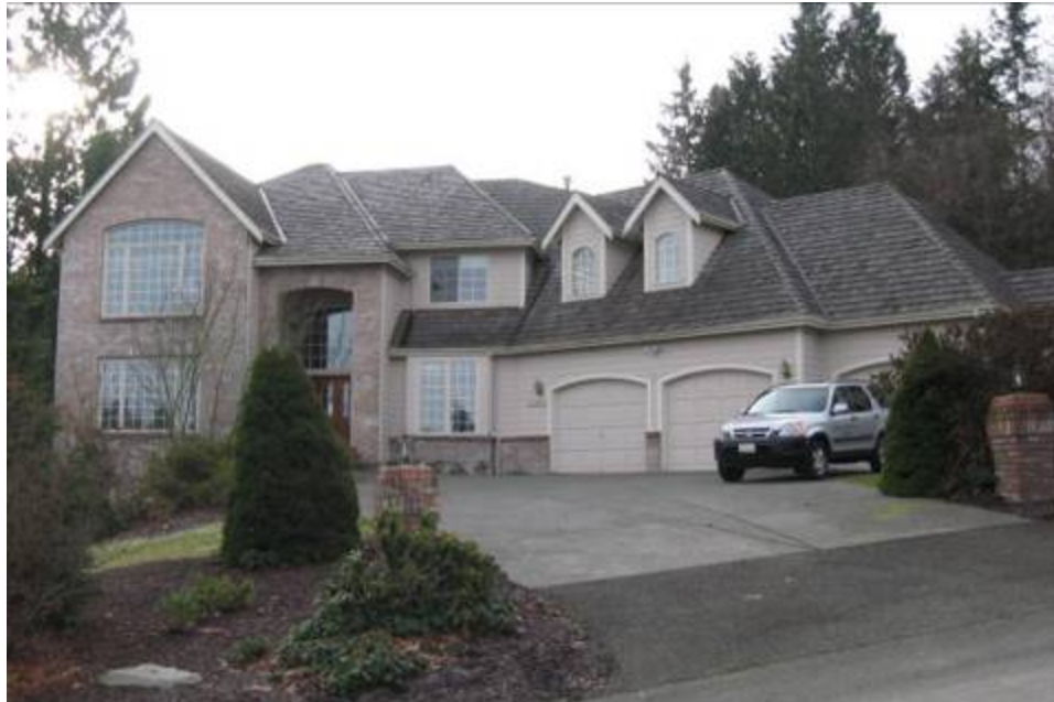
Front View of Inspected Home (Front Faces North)
